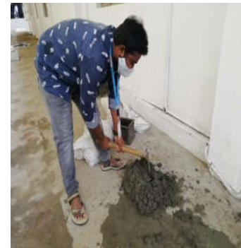
FIG-2.6. MIXING OF CONCRETE
